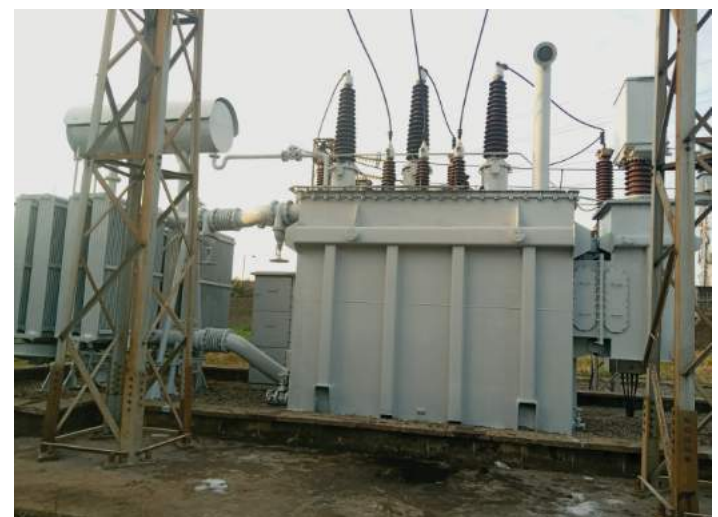
Renovation of 30MVA 132 33kV Transformer at Ijora 132kV Transmission Substation by TCN engineers
