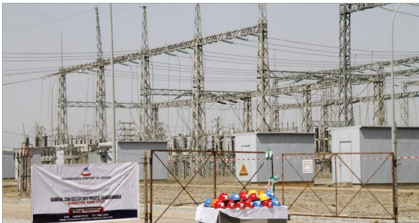
150MVA 330/132/33kV power transformer at Kumbotso Transmission Substation installed by TCN engineers
