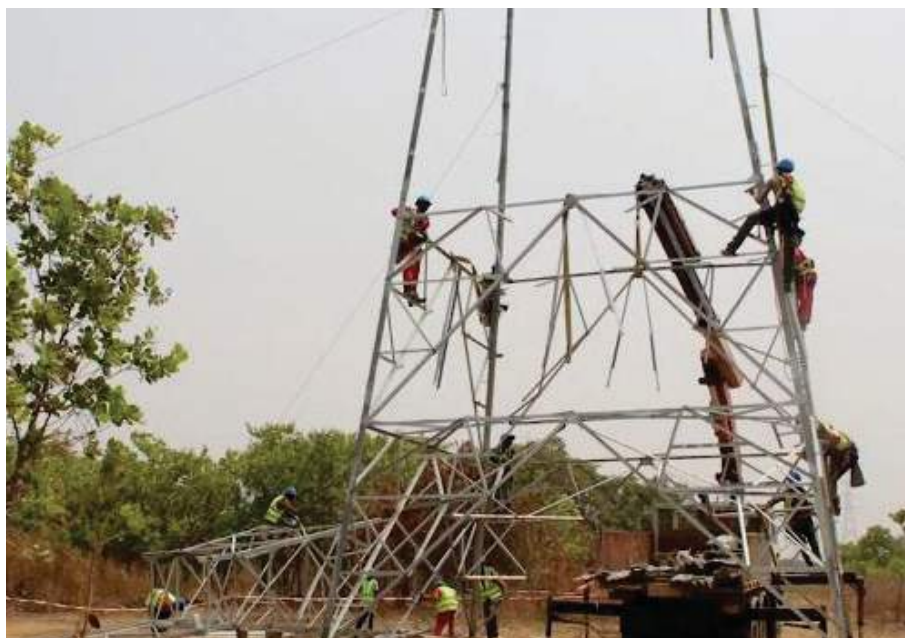
Engineers replacing vandalized tower
