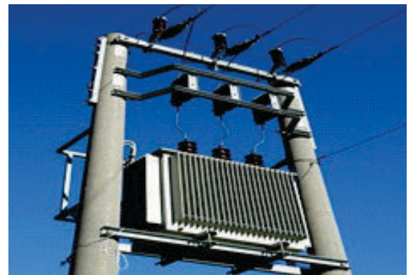
Pole-Mounted Substation
