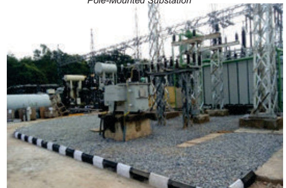
Foundation-Mounted Substation
