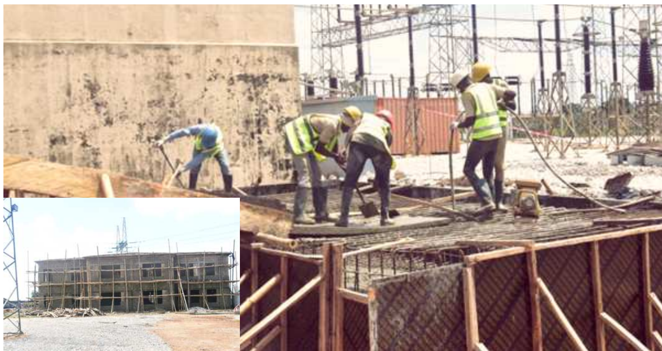
Ongoing work on the plinth of a proposed 4T7 300MVA 330/132kV transformer at Osogbo Sub-Region
