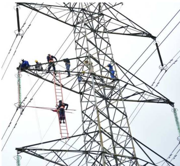
Live Lines crew replacing glass disc insulator with polymersilicon composite insulator
