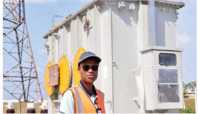
75MX 330kV Shunt Reactor at 330 /132/ 33kV Osogbo Transmission Substation
