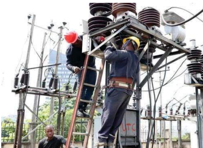
TCN in-house maintenance crew, Port Harcourt Region, replacing faulty red phase 33kV Circuit Breaker pole on UST feeder, at Port Harcourt Town Transmission Substation.
