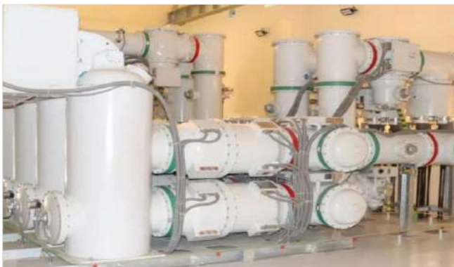
2X60MVA, 132/33kV Gas Insulated Substation (GIS) at Gwarinpa, Abuja
