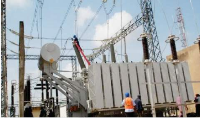
150MVA, 330 /132kV power transformer energized at Ayede Transmission substation
