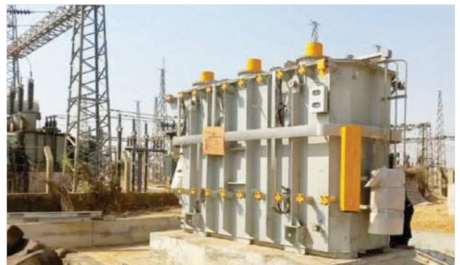
100MVA, 132/33kV power transformer at 132/33kV Dakata Substation, Kano, placed on plinth
