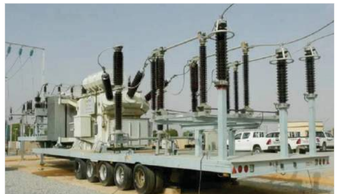
30MVA 132/33kV Mobile Transmission Substation, Bichi
