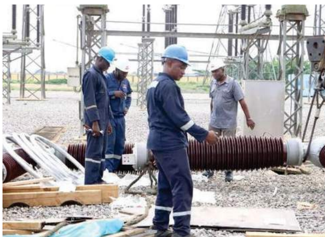
TCN engineers installing 330kV Circuit Breakers at the Ikeja-West 330/132kV Transmission Substation, Lagos
