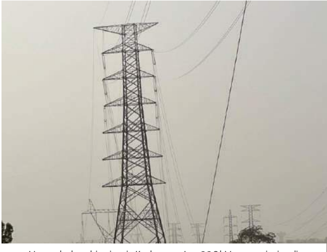
Upgraded multi-circuit Kaduna to Jos 330kV transmission line
