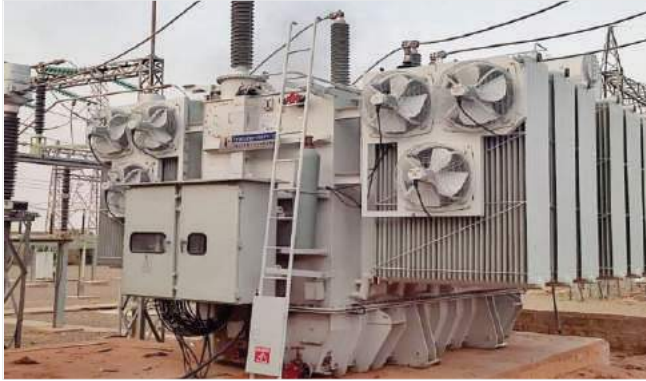
60MVA power transformer in Gombe 132/33kV Substation, installed & energised
