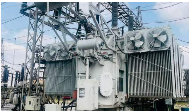
60MVA 132/33kV power transformer at Isolo 132/33kV Transmission Substation, installed and energised
