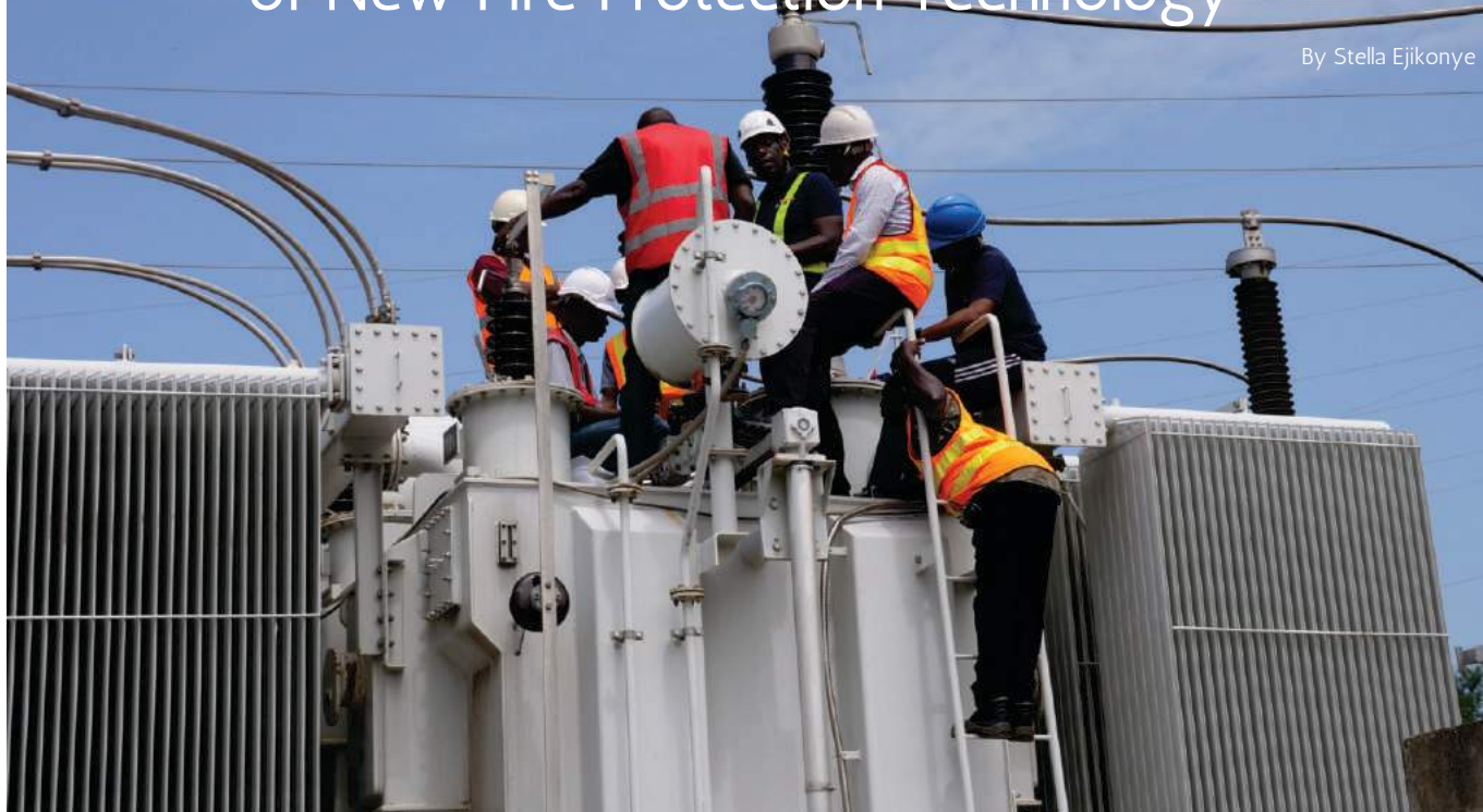
TCN engineers installing a new fire protection system at Katampe 132kV Substation, Abuja
