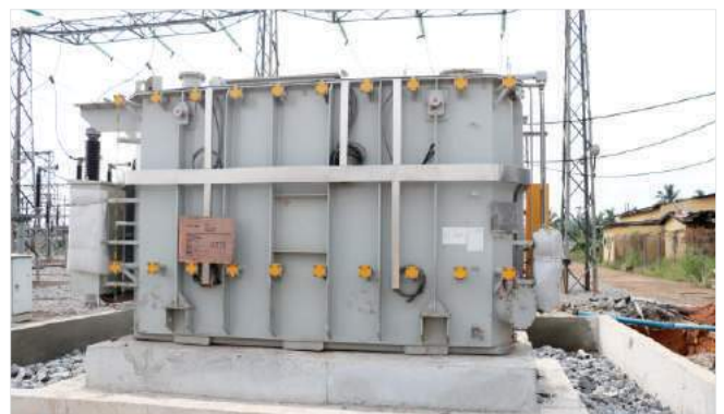
100MVA transformer in Benin sub-region.
