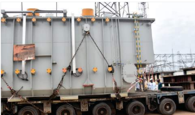
300/375MVA 330/132/33kV power transformer at Osogbo Transmission Substation
