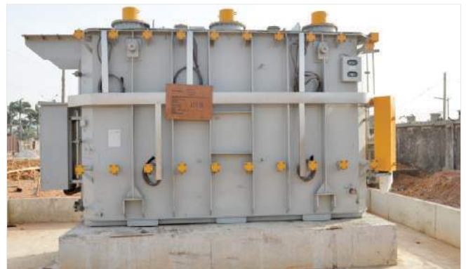
100MVA power transformer at Dan Agundi 132/33kV Transmission Substation
