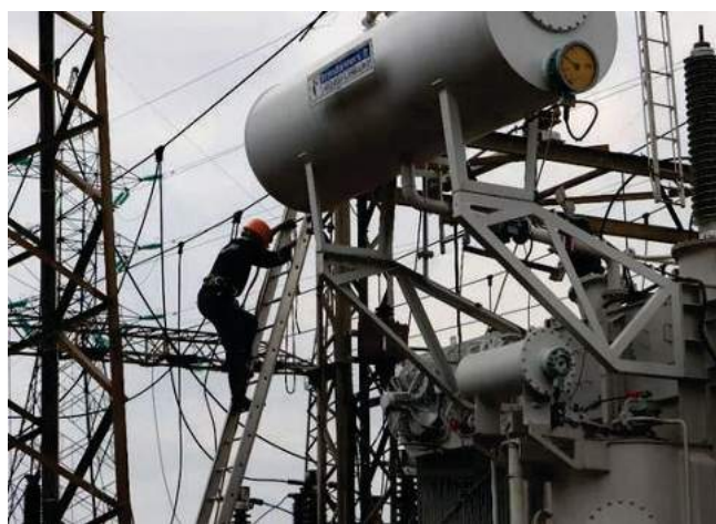
TCN engineers installing 132kV Bus Isolators on 60MVA Transformer T2 at the Isolo 132/33kV Transmission Substation, Lagos State
