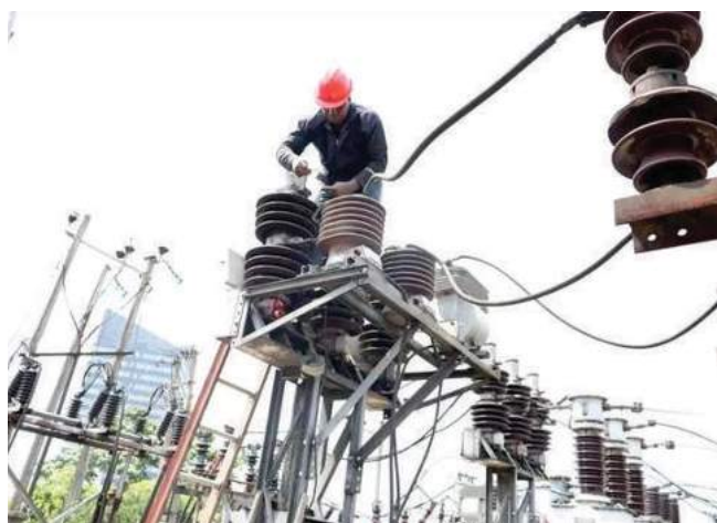
TCN in-house maintenance crew, Port Harcourt Region, replacing faulty red phase 33kV Circuit Breaker pole on UST feeder, at Port Harcourt Town Transmission Substation.
