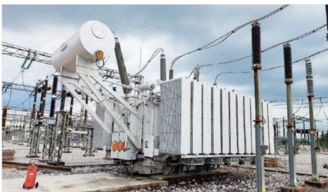
150MVA 330/132/33kV interbus transformer (IBTR) at Delta IV Transmission Substation, installed and energized
