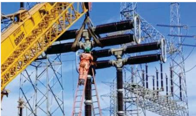
330kV Circuit Breaker installed at Mando 330/132kV Transmission Substation
