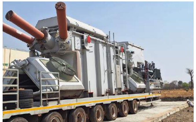
Arrival of 63MVA mobile transformer at Dangora 132/33kV Transmission Substation
