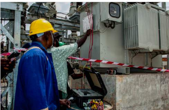
TCN engineers carrying out pre-commissioning test on the transformer
