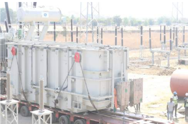
150MVA transformer delivered to 330/132/33kV Bauchi Transmission Substation, Bauchi State
