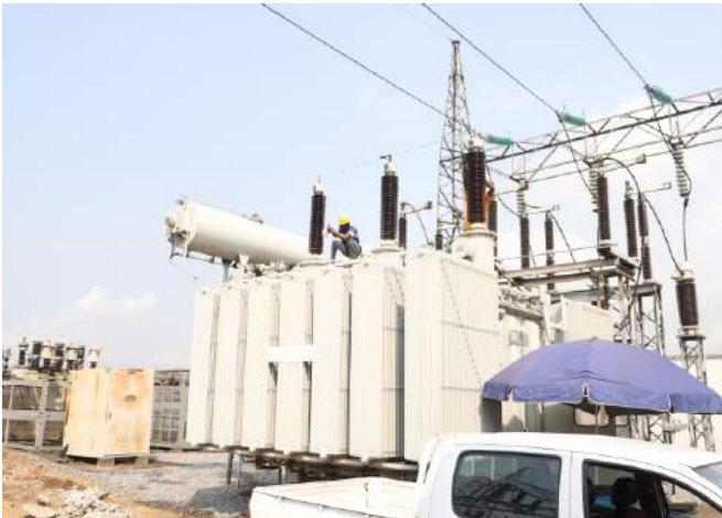
TCN Engineers working on restoring faulty 60MVA 132/33kV power transformer at the Ojo 132/33kV Transmission Substation, Lagos State
