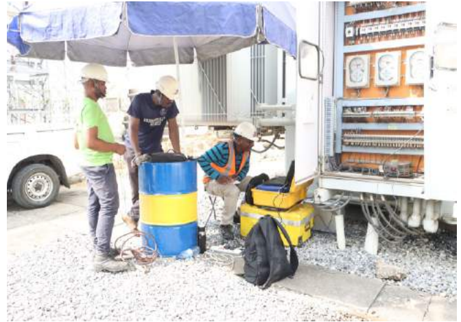
TCN Engineers working on restoring faulty 60MVA 132/33kV power transformer at the Ojo 132/33kV Transmission Substation, Lagos State
