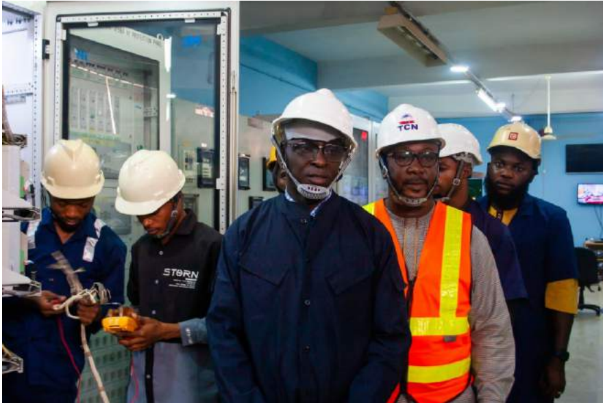
PM Transmission, Engr. Samuel Alade giving report on the panel replacement project
