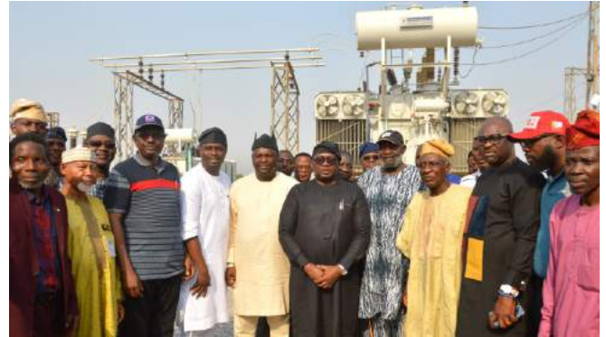
At TCN's new 132/33kV Oyo Transmission Substation in Oluewu Oyo
