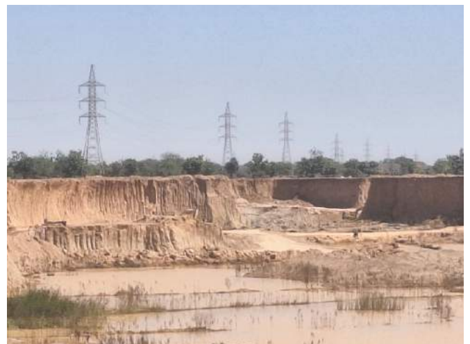
Laterite excavation near TCN transmission towers
