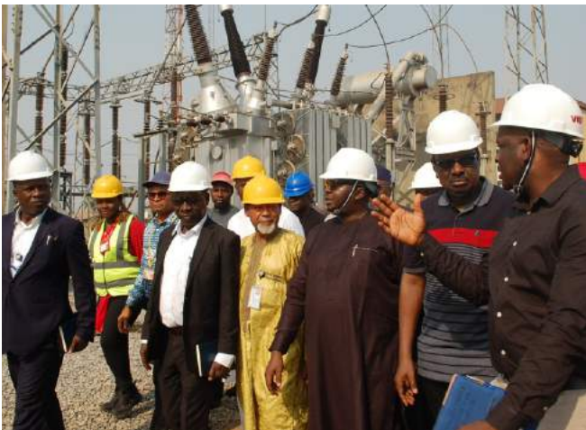
At TCN's 330/132/33kV Ayede Transmission Substation in Ibadan
