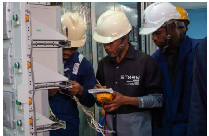
In-house engineers working on SGB TR1 90MVA 330/132/33kV transformer
