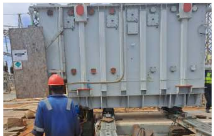
The transformer on plinth
