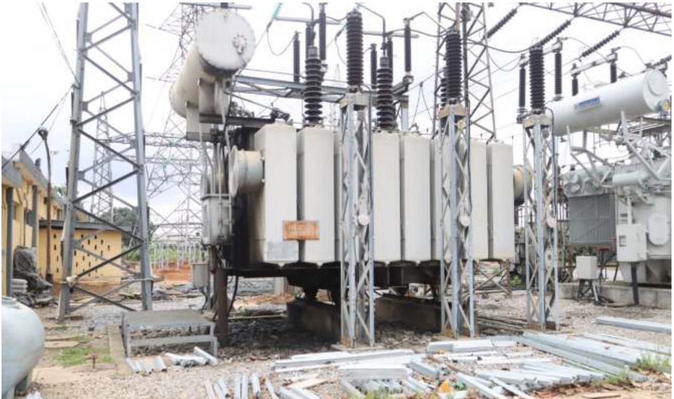
The 60MVA power transformer being upgraded to 100MVA at Isolo Transmission Substation, Lagos State
