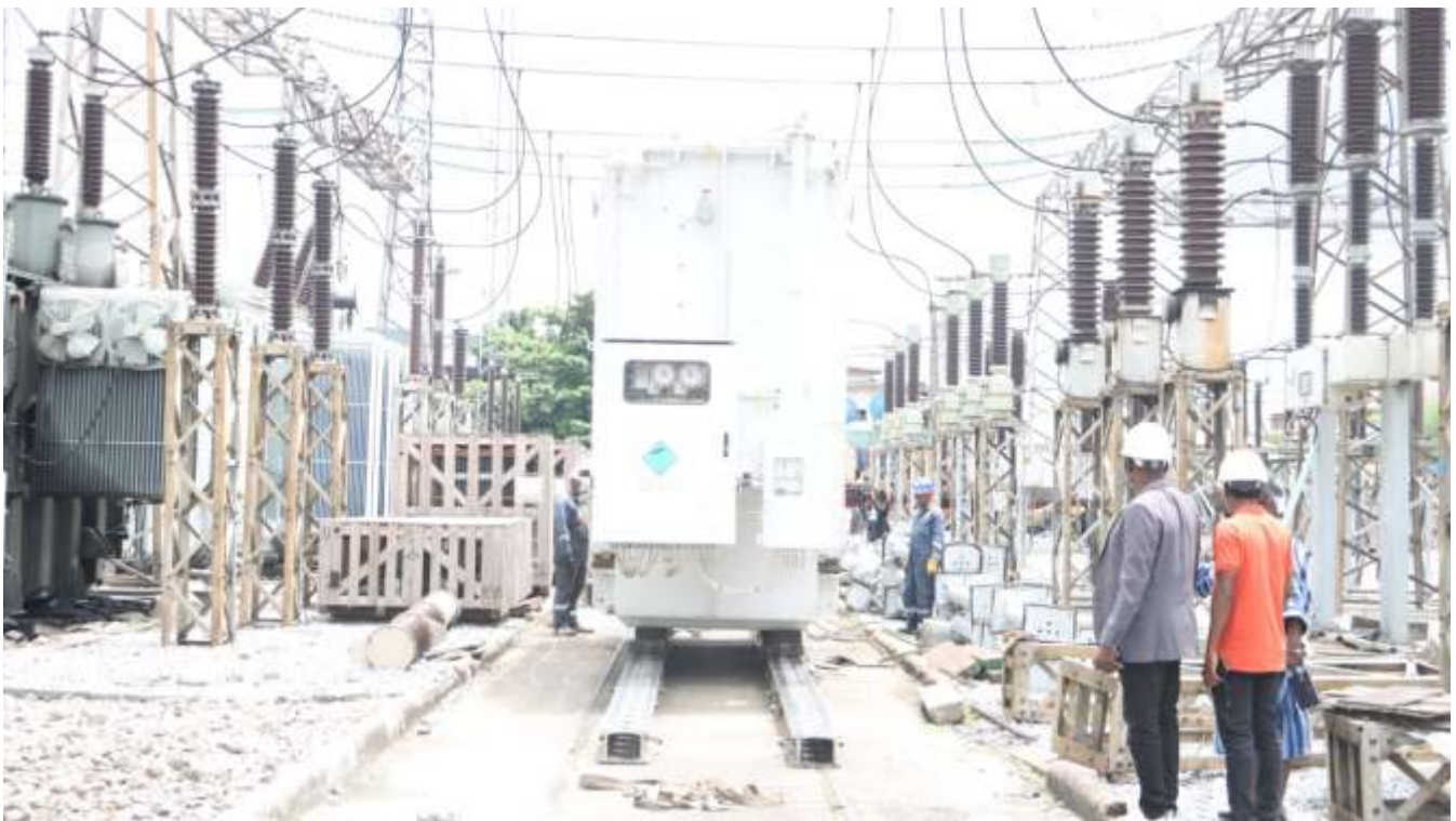
The new 100MVA power transformer at Maryland 132/33kV Transmission Substation
