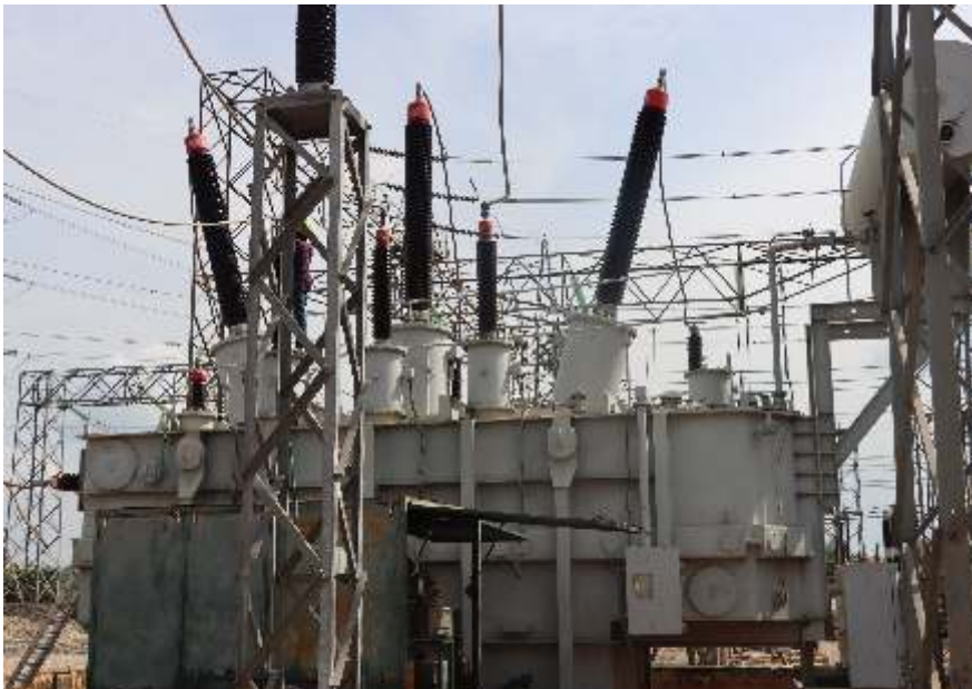
Recently commissioned 150MVA, 330/132kV power transformer at New Haven, Enugu State
