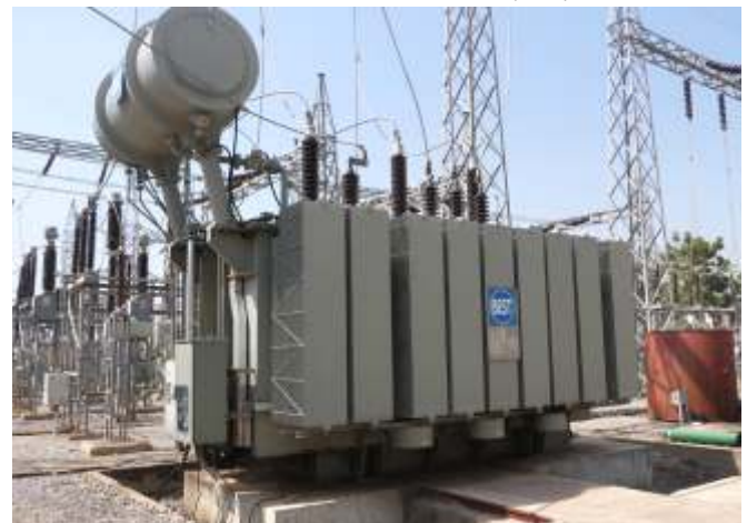
Installation of 60MVA power transformer by TCN engineers at 132/33kV Kubwa Transmission Substation
