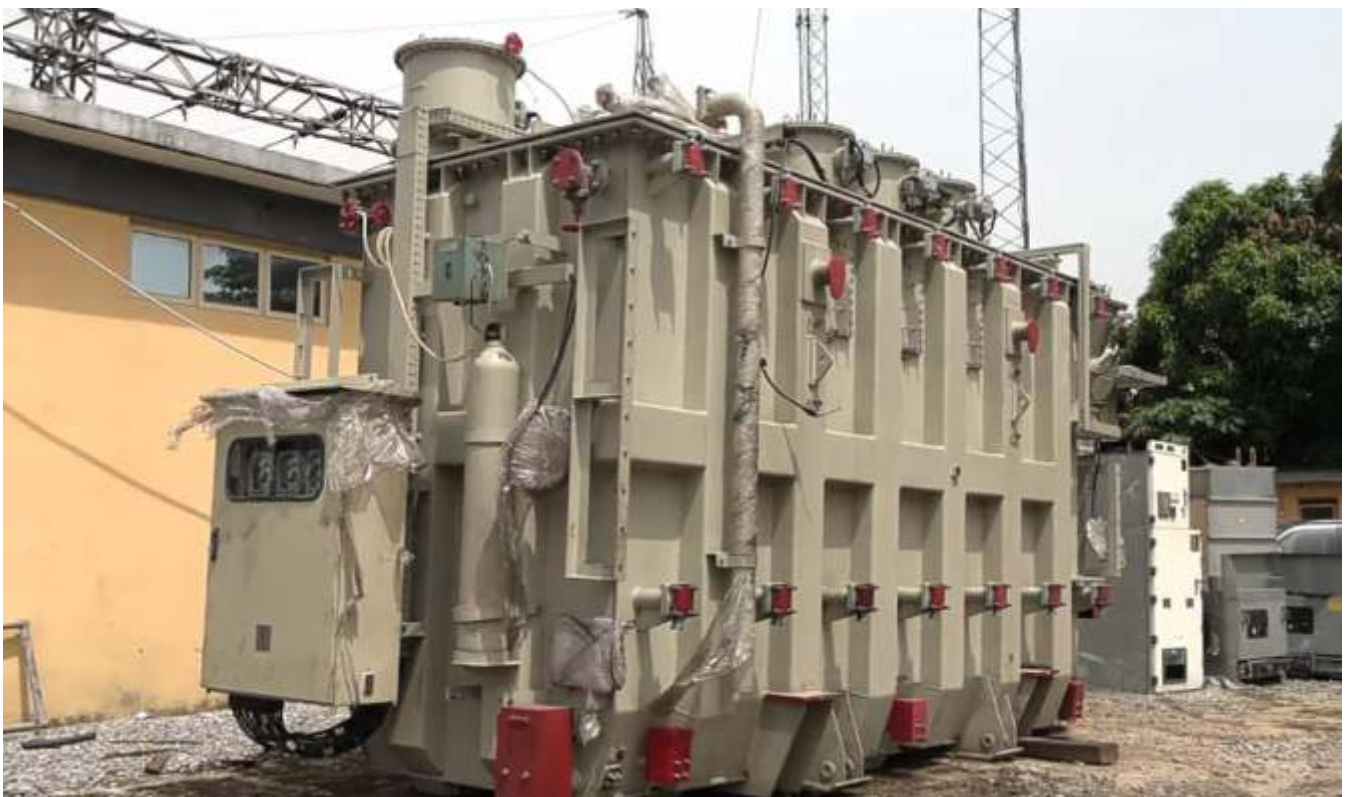
The new 60MVA power transformer at Oworo 132/33kV Transmission Substation, Lagos State
