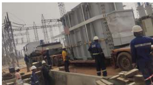
Installation of 100MVA transformer at Birnin kebbi Substation
