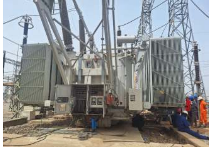
Energization of newly installed 150MVA power transformer in 330/132/33kV Kumbotso Substation in Kano, on Thursday, November 23, 2023. With the commissioning of the new transformer, TCN has added 120MW to the substation capacity
