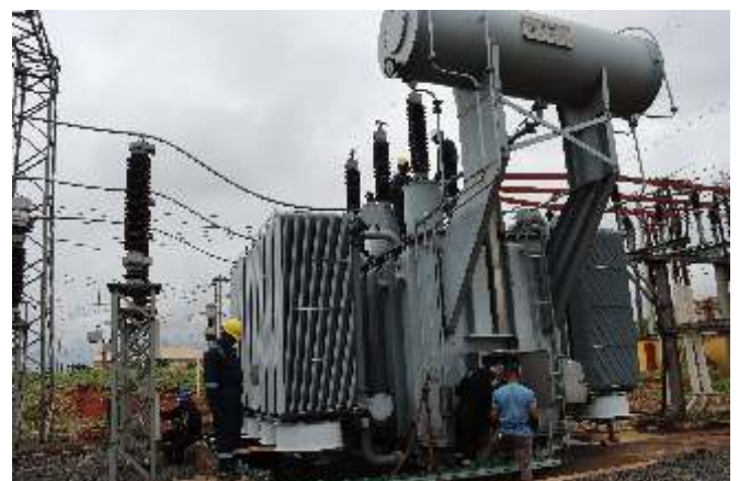
The new 100MVA 132/33kV power transformer at Onitsha Sub-region
