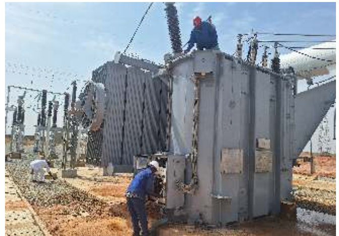
TCN Kano Region energized a new 40MVA 132/33kV power transformer at its Bichi Transmission Substation on Sunday, November 26, 2023. The 40MVA transformer, which replaced the 20/30MVA 132/33kV Mobile Transformer in the substation, added 32MW to the capacity of the substation
